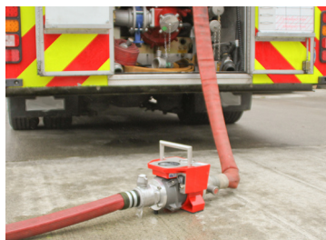
Fig. 1.4 Testing a fire pump
