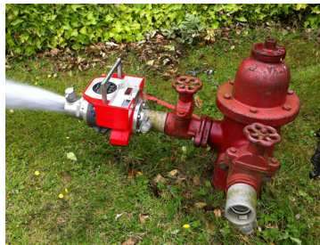
Fig. 1.3 Testing a pillar fire hydrant on a high pressure ring main
